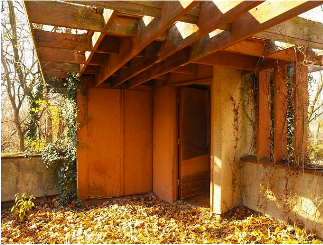
Tower rooftop trellis and outdoor Murphy bed Photography credit: Tom Hogan
